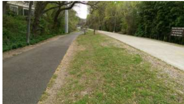
The Katy: main concrete section (r) and rubberized running/walking section (l)
